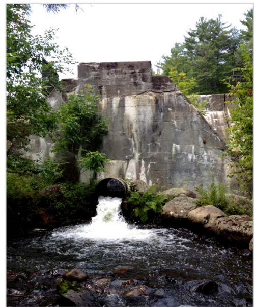
Kingdom Dam Outlet
