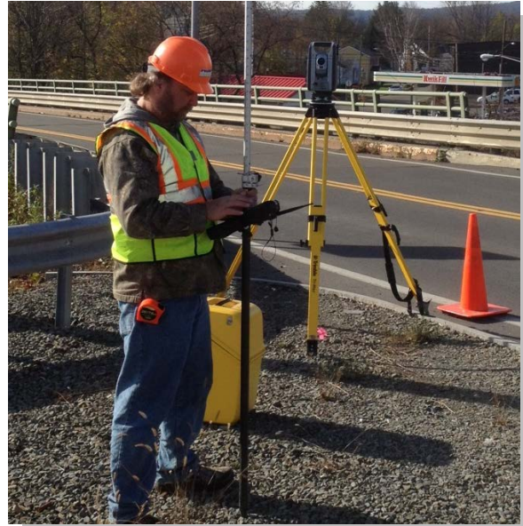
Collecting topographic data at Hooper Road Bridge
