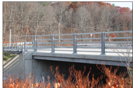
New Connection Road Bridge Deck
