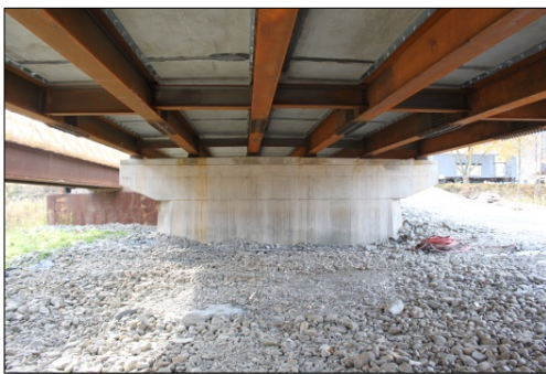
NYS Route 960H Bridge
