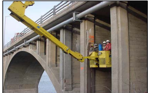
NYSDOT Region 3 - Minetto Bridge Inspection, Minetto, New York
