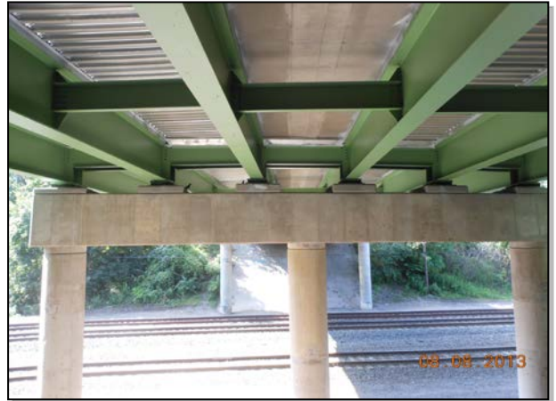
Costello Parkway (CS55) over CSX Railroad
