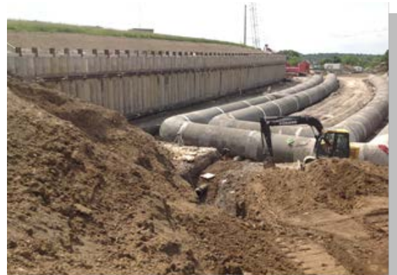
Excavation Support Wall and Bypass Piping Area
