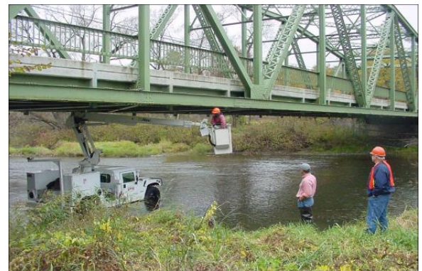
NYSDOT Region 9 - Unadilla River
