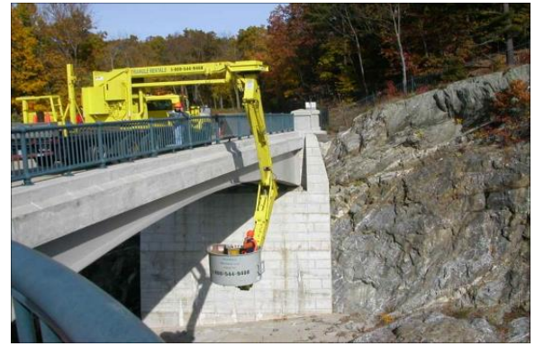
NYSDOT Region 8 - Cross River Reservoir
