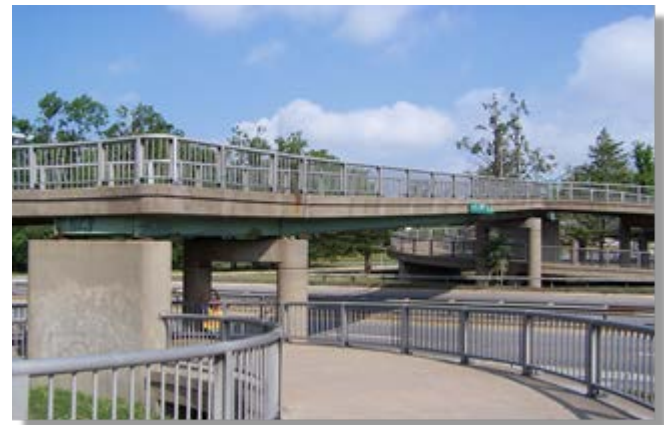
Pedestrian Bridge over Scajaquada Expressway
