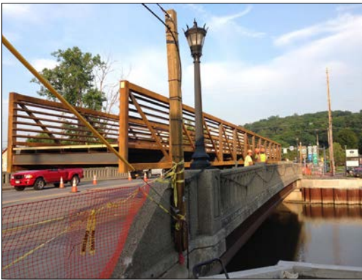
Cayuga Trail Pedestrian Bridge Ready for Placement Over the Canal
